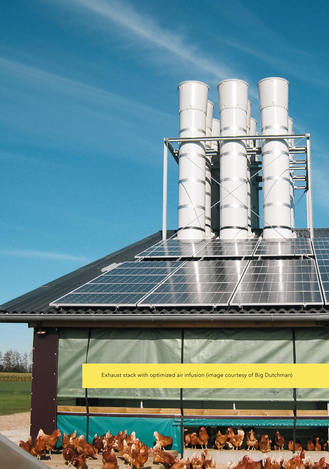
Exhaust stack with optimized air infusion (image courtesy of Big Dutchman)
